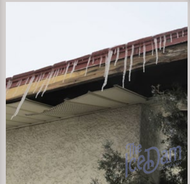
SOFFIT DAMAGE
