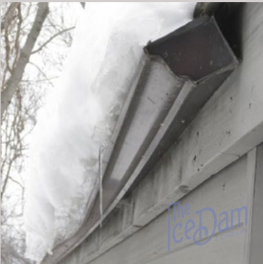
GUTTER DAMAGE
